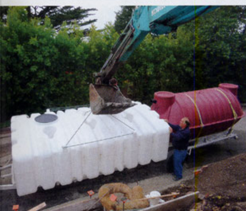
Ready for the rain barrel. Domestic water needs are partially supplied by rainwater stored in this 2500-gal. tank.
